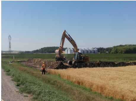
Aug 21/18 Photo facing South West SF 30 access Top soil stripping & Grader grading ROW
