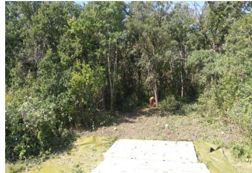
Aug 21/18 SF 31 (KP 961+025) Photo facing West Chainsaw operator falling tree
